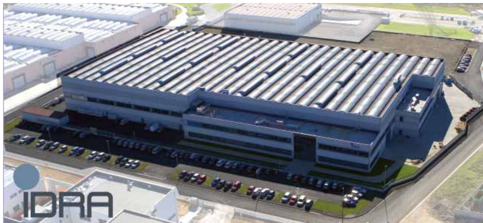
Idra's plant in Italy
